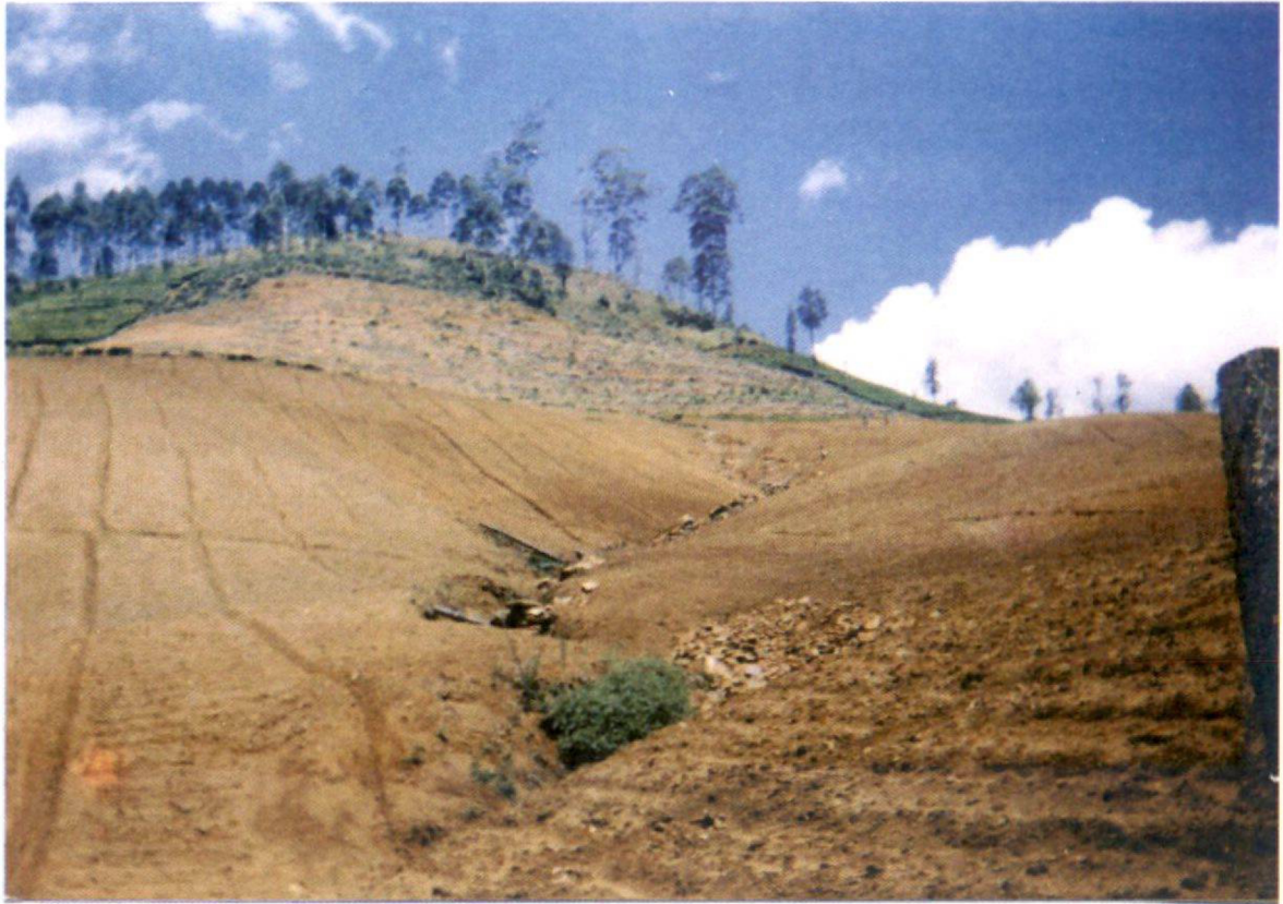
Fig. 13 Soil Erosion on Steep Slopes
