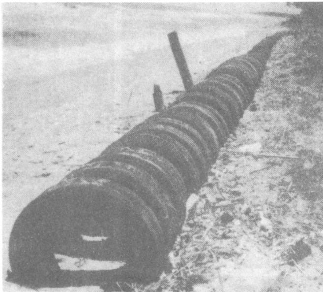
Tyre barrier mounted on the shore behind which eroded sand has accumulated.
