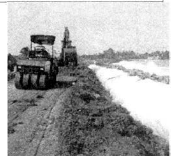
Maintenance of 1km Revetment at Akurala.
