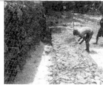
Gabion Revetments at Induruwa (150m).
