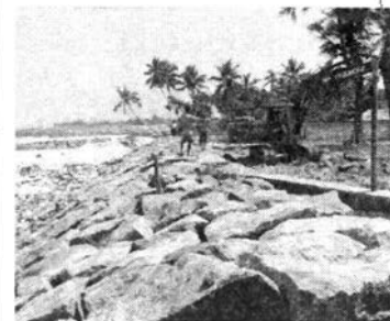
100m Revetment at Patabadimulla
