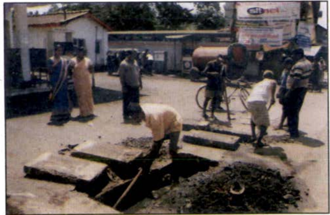
Drain system in Negombo MC area rehabilitated Under Beauty City Programme
