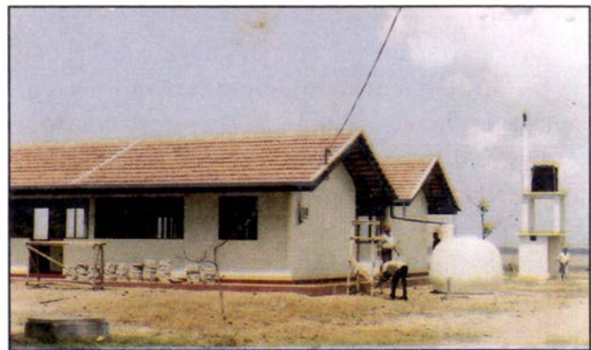
Eco village was constructed with the support of fishing community under Tsunami rehabilitation programme in Kahadamodara
