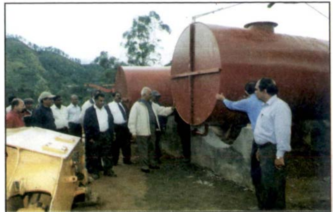
A new impregnation plant installed at Kappetipola
