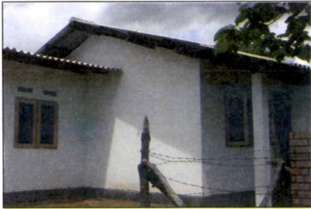
Building constructed for the site office and stores for Solid Waste Management Project Gallaella
