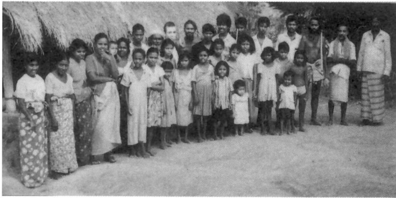
The future wardens of the new settlements with their elders
